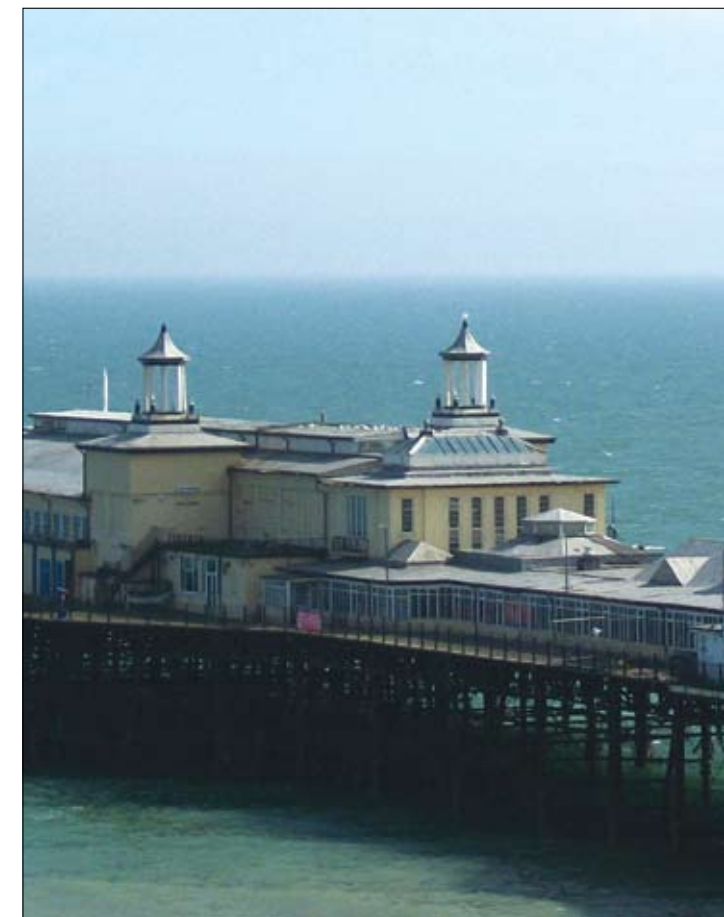
Hastings Pier Photograph Amy Searle
